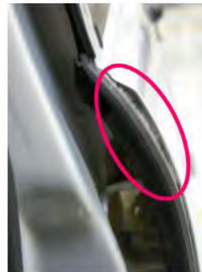
Bad fixture sealing part !!
